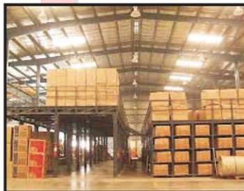
SLOTTED ANGLE MEZZANINE FLOOR
